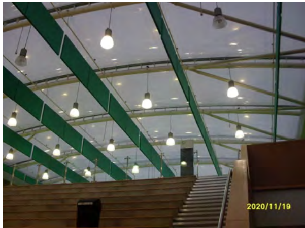
General view of ETFE roof and gallery
