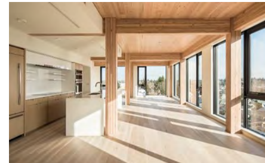
Figure 3 CLT Frame
