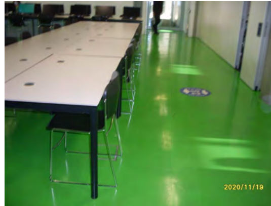
General view first floor vinyl
