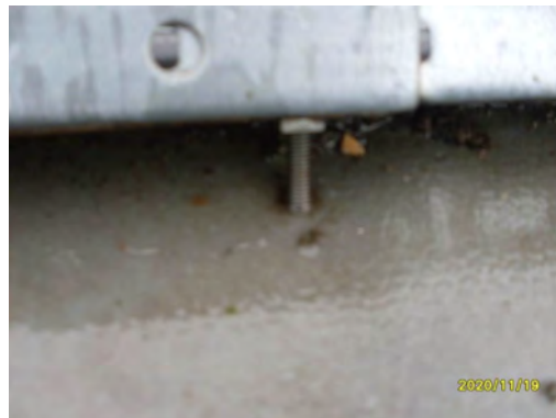
Screw from tray touching the membrane
